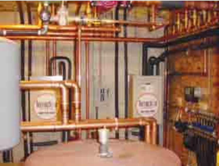
Two (of four) hot water exchangers and a water storage tank make up this hydronic heating system.
