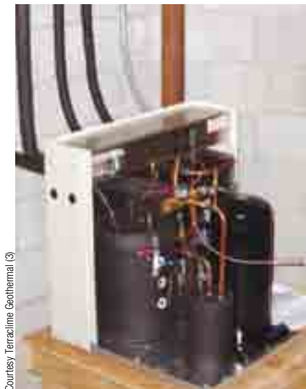
The inner components of a ground-source heat pump.
